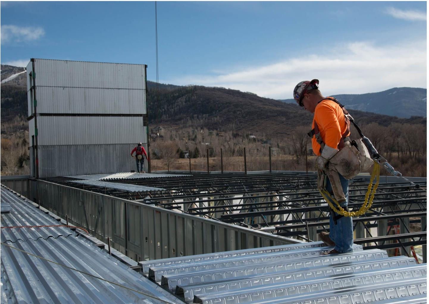
**“ The overall composite design eliminates shoring and allows for open spans, all while using a thinner slab. That saves head room and makes clients happier.”**
